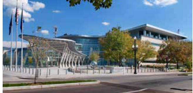
Salt Lake City Public Safety Building: Critical equipment is protected by an extensive DIS Isolated Platform System.
