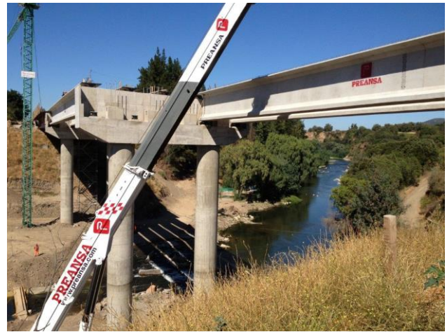
Figure 03: Base isolated replacement Rio Claro Bridge, Chile
