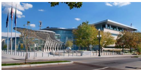
Figure 20: The Salt Lake City Public Safety Building (SLC PSB)
