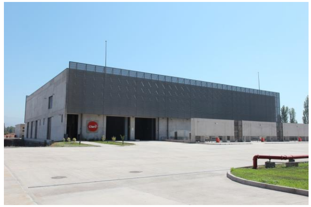
Figure 07: Claro Data Center, Chile
