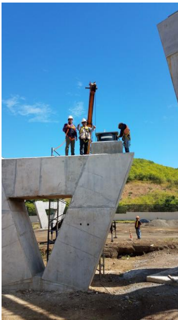
Figure 12: Construction of the first base isolated bridge in Nicaragua
