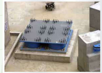
Groups of four isolators are located under heavily-loaded columns in the Tan Tzu Medical Center.
