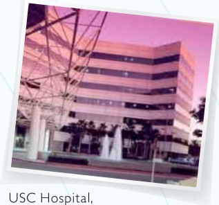
USC Hospital, Los Angeles, California.
