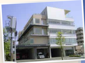
The Funabashi Fire Station is one of many fire stations in Japan that are base isolated.
